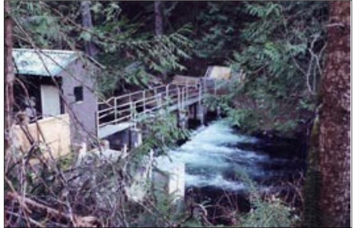
The dam on Sakinaw Creek controls the lake level and enables Fisheries employees to count salmon. Daniel Bouman photo
